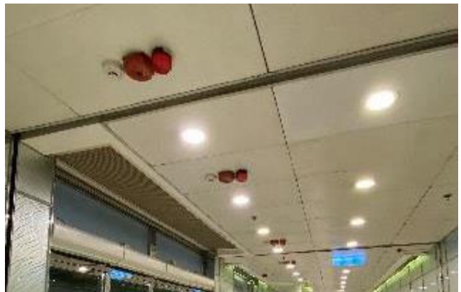
“巴士附近有多個火警鐘在顯眼位置” “Fire alarms near bus stop are clearly visible”
